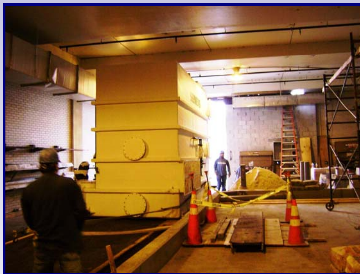
Asbury Park WWTP—Asbury Park, NJ (2009)
