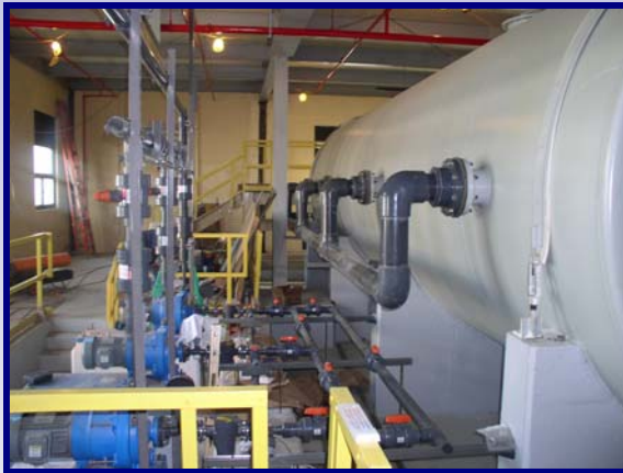
Belmont WWTP—Philadelphia, PA (2006)
