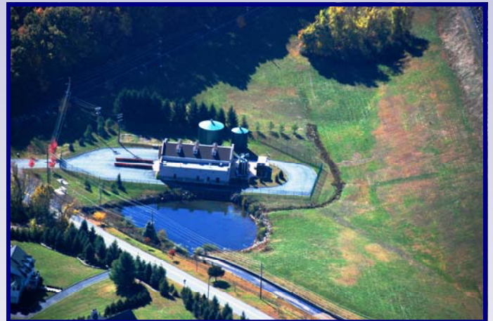
Clyde Potts Membrane Filtration Plant—Mendham, NJ (2004)
