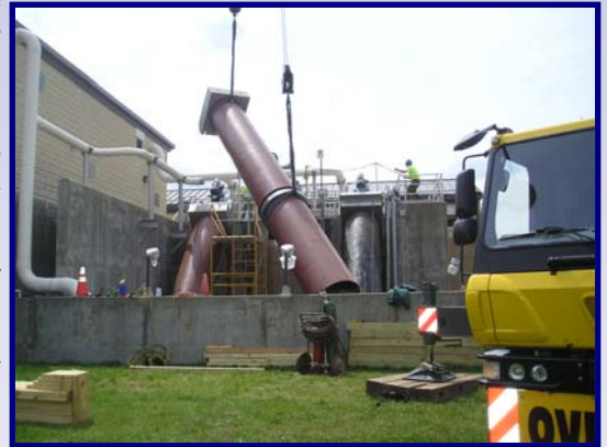
New pump begins descent into its final resting position
