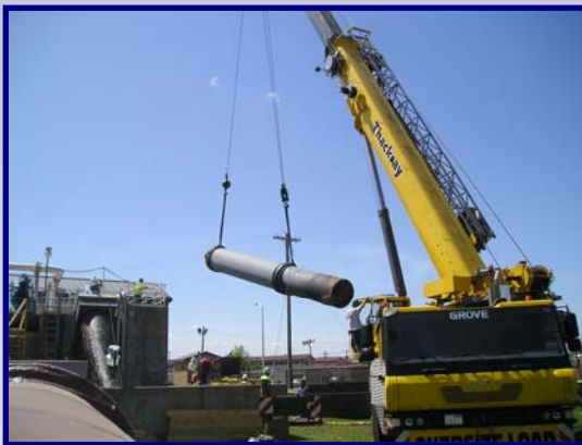
Stone Hill and Thackray Crane Service remove old screw pumps
