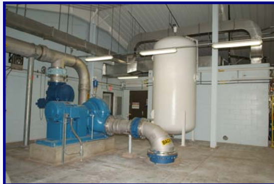
Interior of Filter Building
