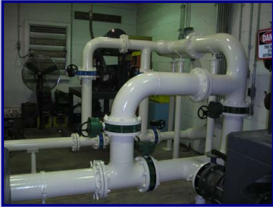
Aeration Pipe Additions for Tank T-5
