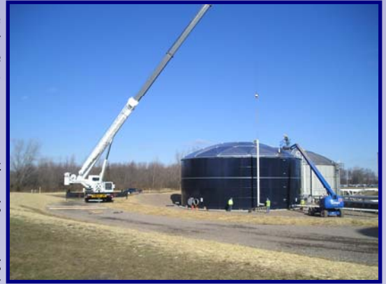
Stone Hill Crew Installing Final Tank Piping
