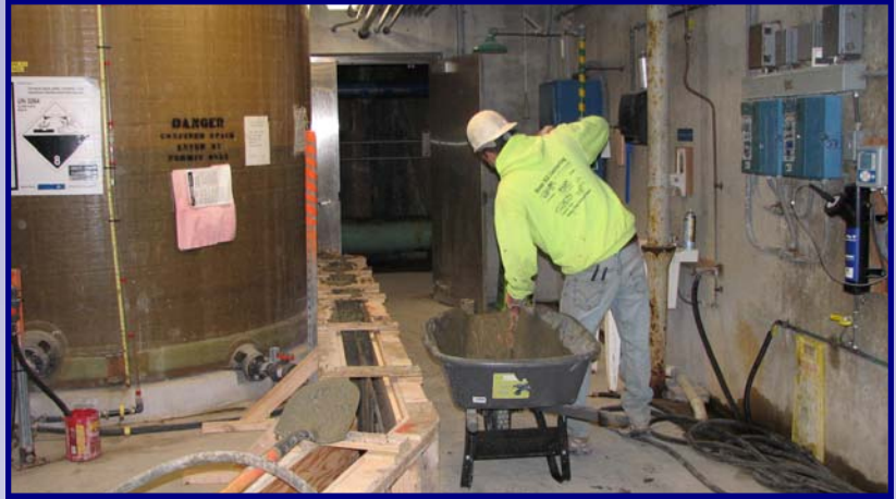
Pouring the Containment Curb at the Existing Chemical Building
