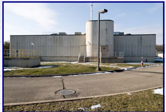
Existing Site at Two Bridges WWTP
