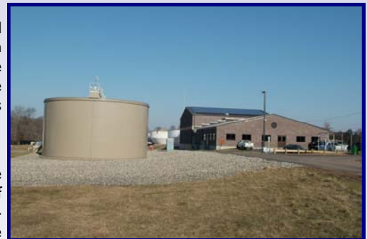
Filter Building and Gravity Feed Tank
